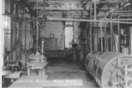
Fullarton Refuge Infirmery and Fullarton Refuge Wash House undated, Courtesy Adelaide Catholic Archdiocesan Archives.
